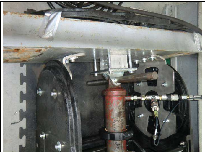
bended brackets pull test 16.06.11
